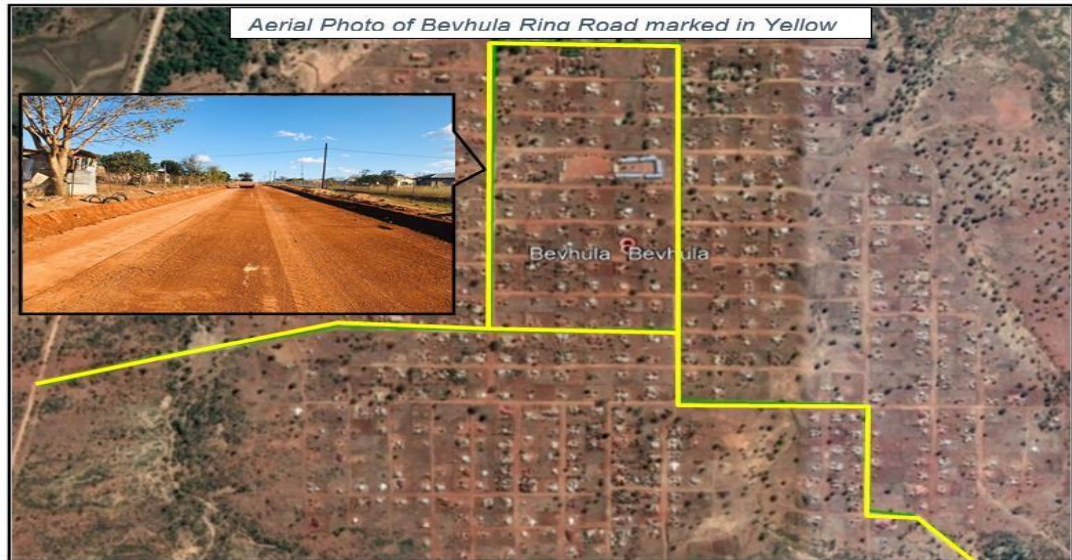
Picture 8 Upgrading of Bevhula Ring Road.
