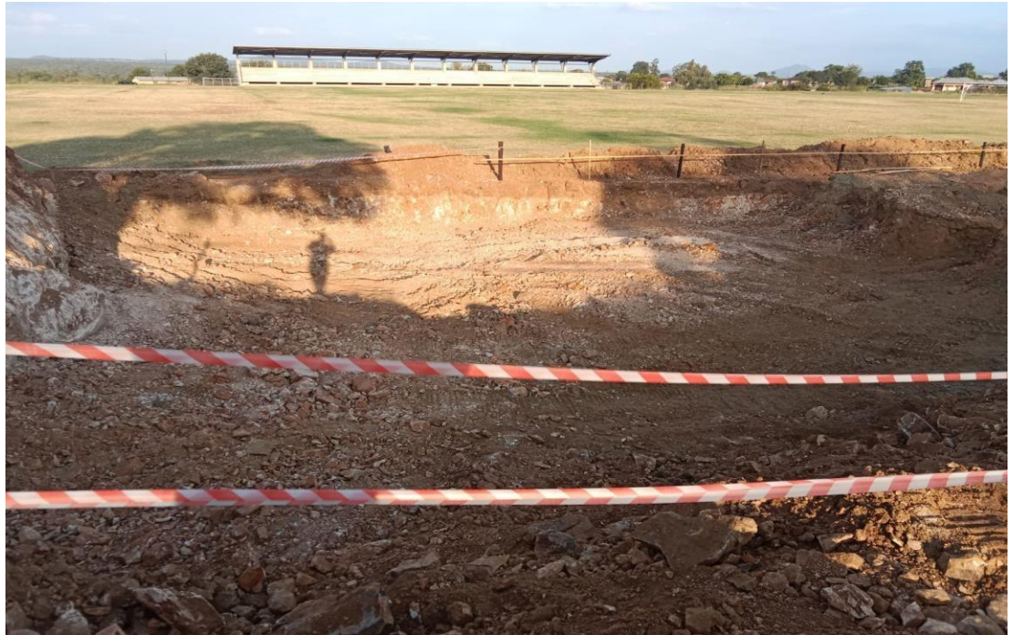
Picture 13 Construction of Davhana Stadium Phase 1
