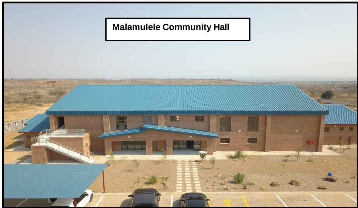
Construction of Malamulele Community Hall
