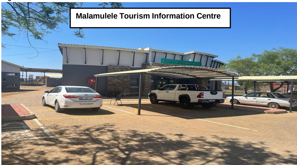
Construction of Malamulele Tourism Information Centre
