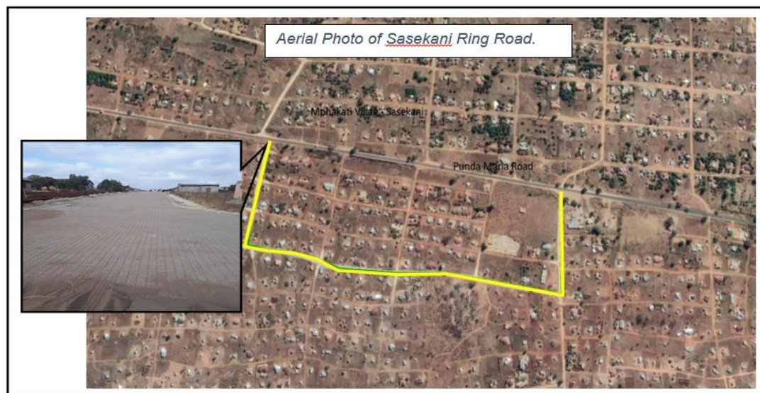
Upgrading of Sasekani Ring Road
