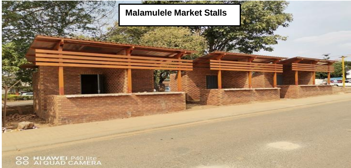
Construction of Malamulele Market Stalls
