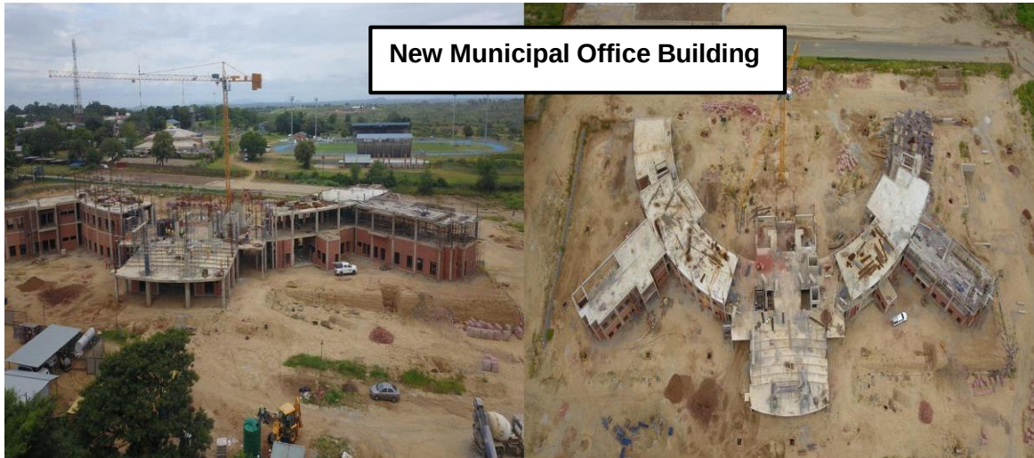
Construction of New Municipal Office Building
